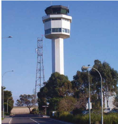
Melbourne Air Traffic Control Tower
