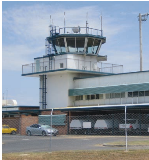
Rockhampton Air Traffic Control Tower
